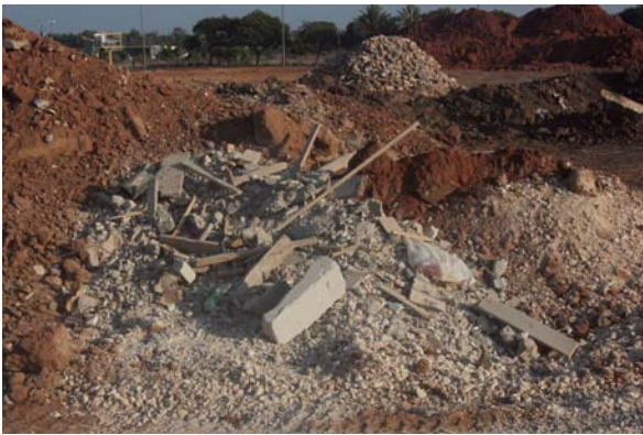
ABOVE Construction, Herzliya, Israel
